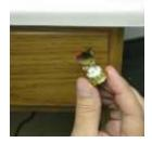
Locate the sensor wire from the top of the pump, (see picture below), and the white plastic end connector. This will need to be connected to the connector from the D'MAND KONTROLS<sup>®</sup> controller box. This will allow your pump to sense water temperature differential in the water line.
