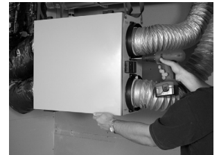
Fix and secure with four screws supplied and seal all joints.
