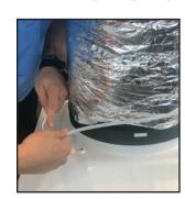
Use second duct strap to secure insulation
