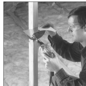
Attach Mounting Bracket to stud using screws provided.
