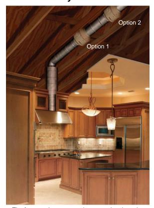
The fans can be connected at any point along the ventilation duct: along the duct or at the end.
