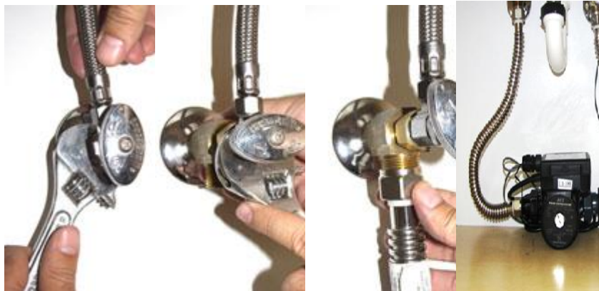
1. Turn off water supply and remove angle stops.
