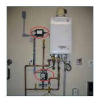
2. Under Sink Installs at the furthest fixture where no loop or return line is available - Requires power
