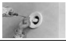
1.2 Using the appropriate hole cutting tool, cut a 4-1/8" diameter hole through the siding, sheathing, insulation and interior wall surface. Be careful to properly align the holes on the interior surface with the exterior, and ensure a slight slope towards the outside.
