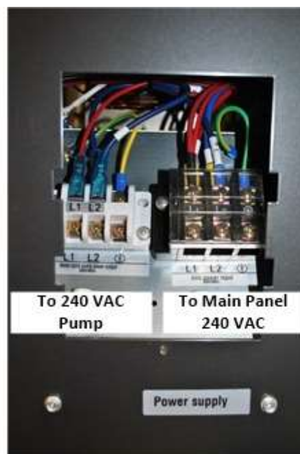
Connect Main & Pump power
