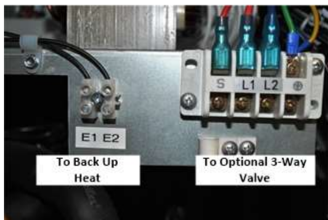
Remove front panel to access accessory Terminal Blocks
