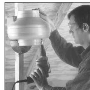
Attach Fan to Mounting Bracket using screws provided.
